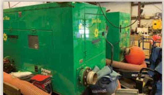
Two six-inch pumps are on-hand to respond to significant flooding events.
