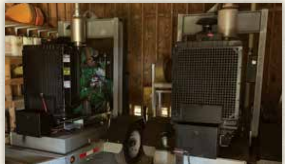
Two 4-inch diesel pumps are available to respond to major flooding.
